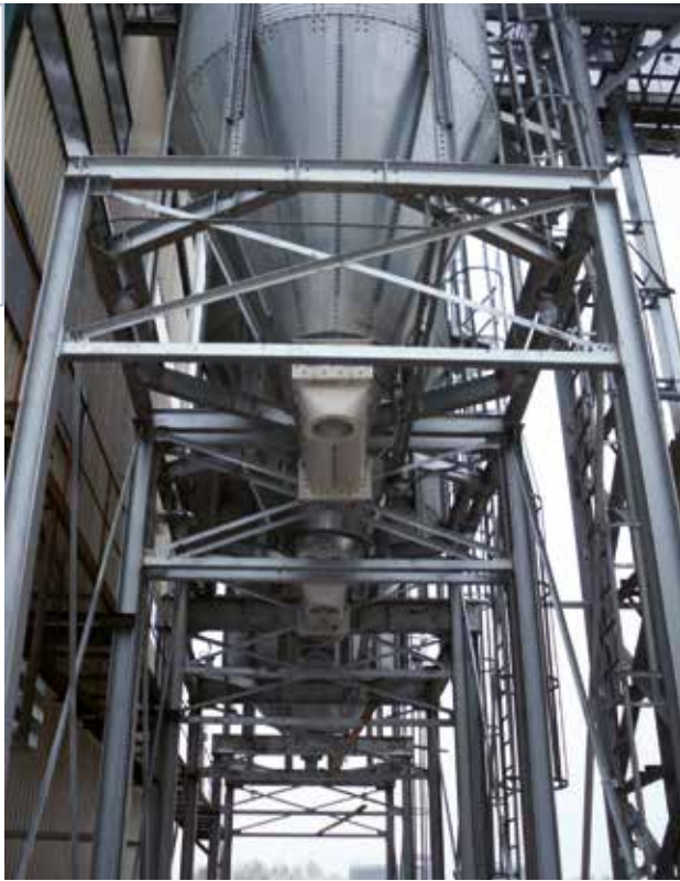
SUPPORT STRUCTURE FOR DELIVERY SILO
